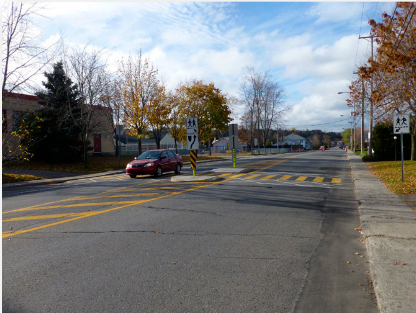
Figure 30 : îlot refuge, 2 e rue, Rimouski
